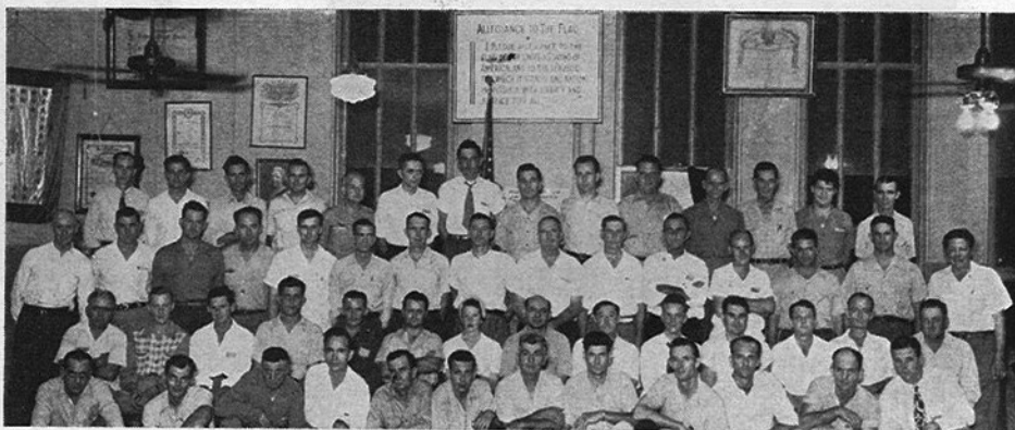
Refrigeration Fitters of Houston, Texas, Initiated Into L. U. No. 195
