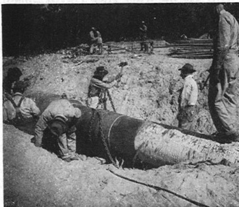
Final Test and O. K. of Joint
