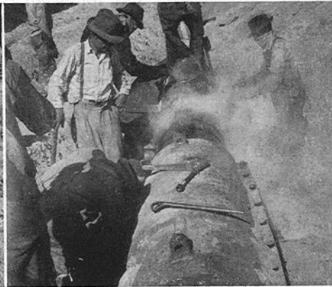
Placing River Sleeve Over Weld
